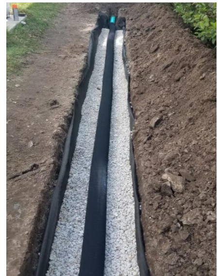
Installation of a French drain
